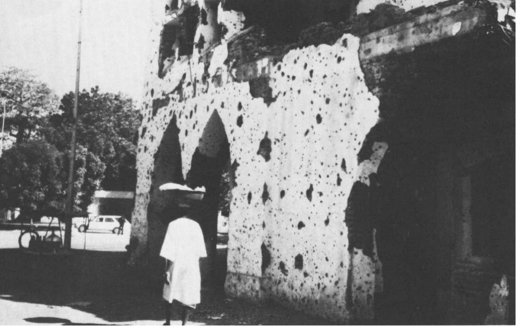
A building showing the destructiveness of the Chadian Civil War Courtesy United Nations (John Isaac)
